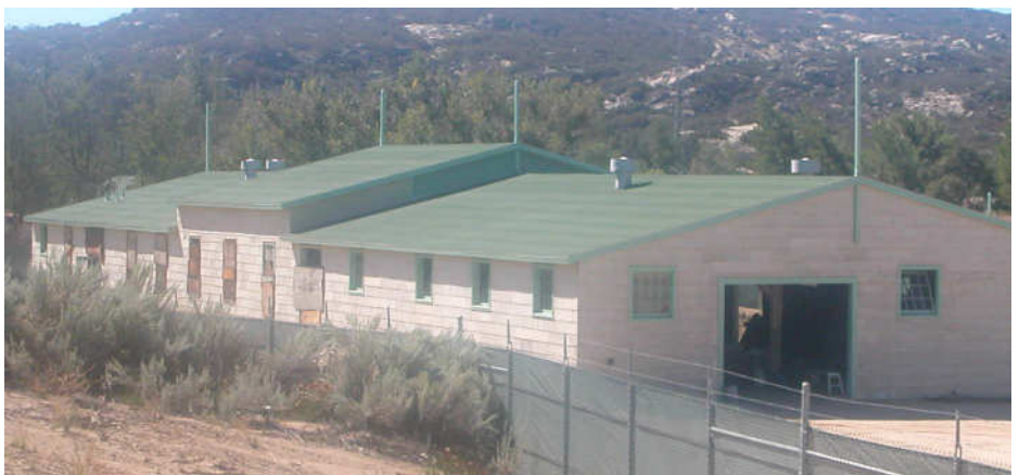
A new roof and repainted windows improve this stable building’s appearance
