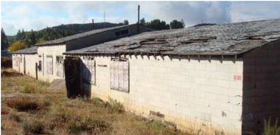
Deterioration of the roof can be seen on this stable building before reroofing.
